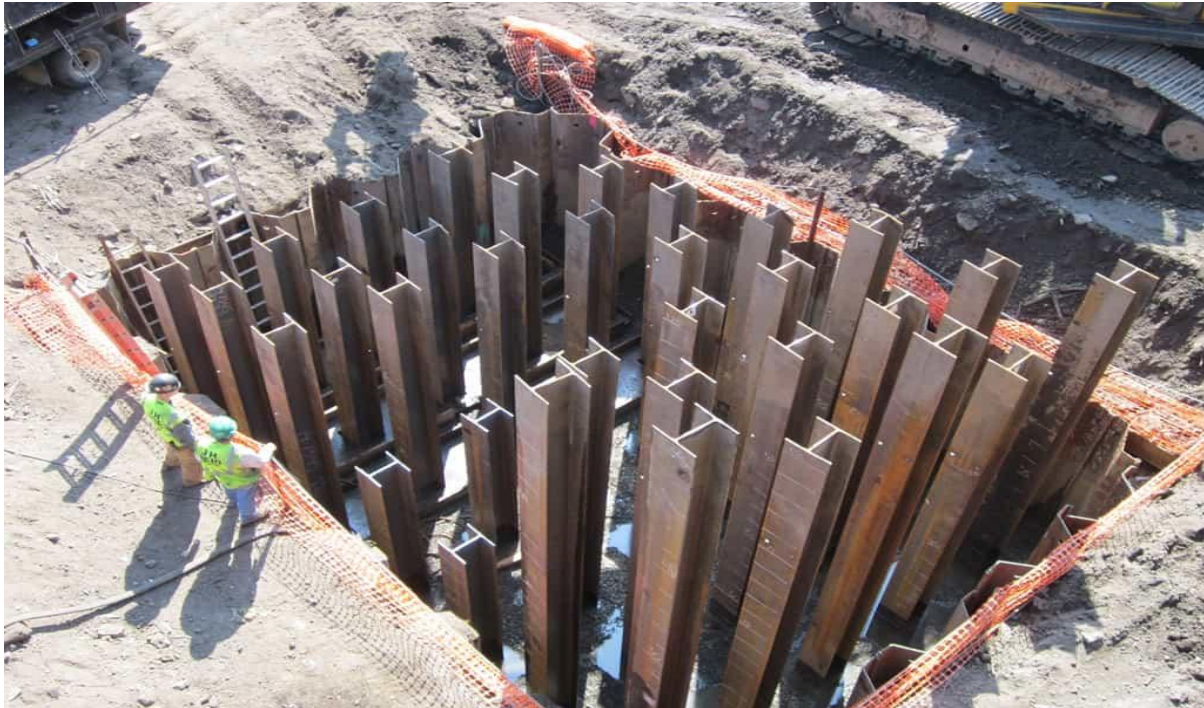
Installation of steel piles
